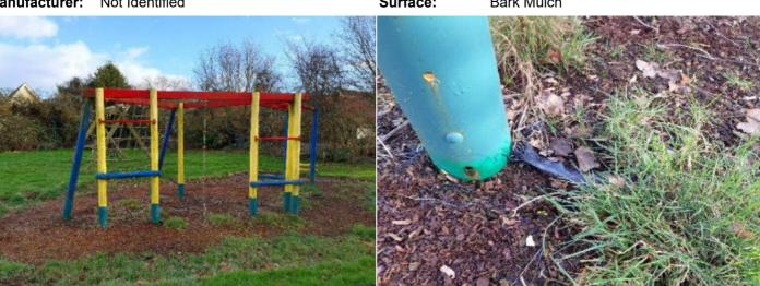
Finding: The safety surface is low and the membrane is exposed creating trip points
