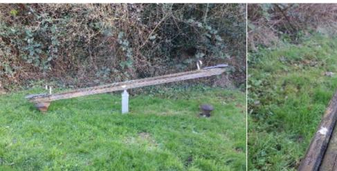
Finding: The timber has a number of splits/shakes or air Action: Monitor to ensure the splits do not cross through cracks and this may affect the stability or allow water ingress fixing points of the structure and/or cause any instability which will accelerate the rotting process
