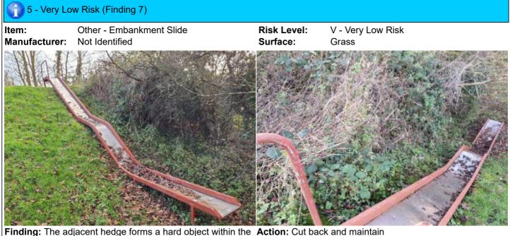
**Finding:** The adjacent hedge forms a hard object within the **Action:** Cut back and maintain free space of the equipment in contravention of the requirements of BS EN 1176 Part 1
