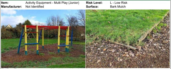
Finding: There are areas or parts of the timber edging that Action: Replace all affected timbers have rotted or are damaged
