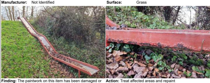
worn exposing the metal underneath which is rusting / corroding
