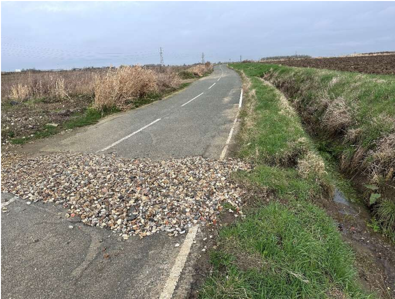
- Land drain on mill lane
